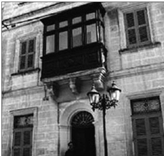
Building House from the Paolo Freire Institute in Zejlun Source: Peter Mayo
