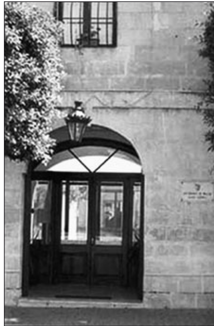
Building House from the Paolo Freire Institute in Zejlun Source: Peter Mayo
