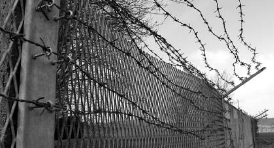
Border fence at the border memorial Gompertshausen, Thuringia
